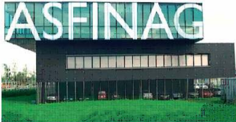
Figure 6 – ASFINAG Traffic Management and Information Centre (TMIC)
