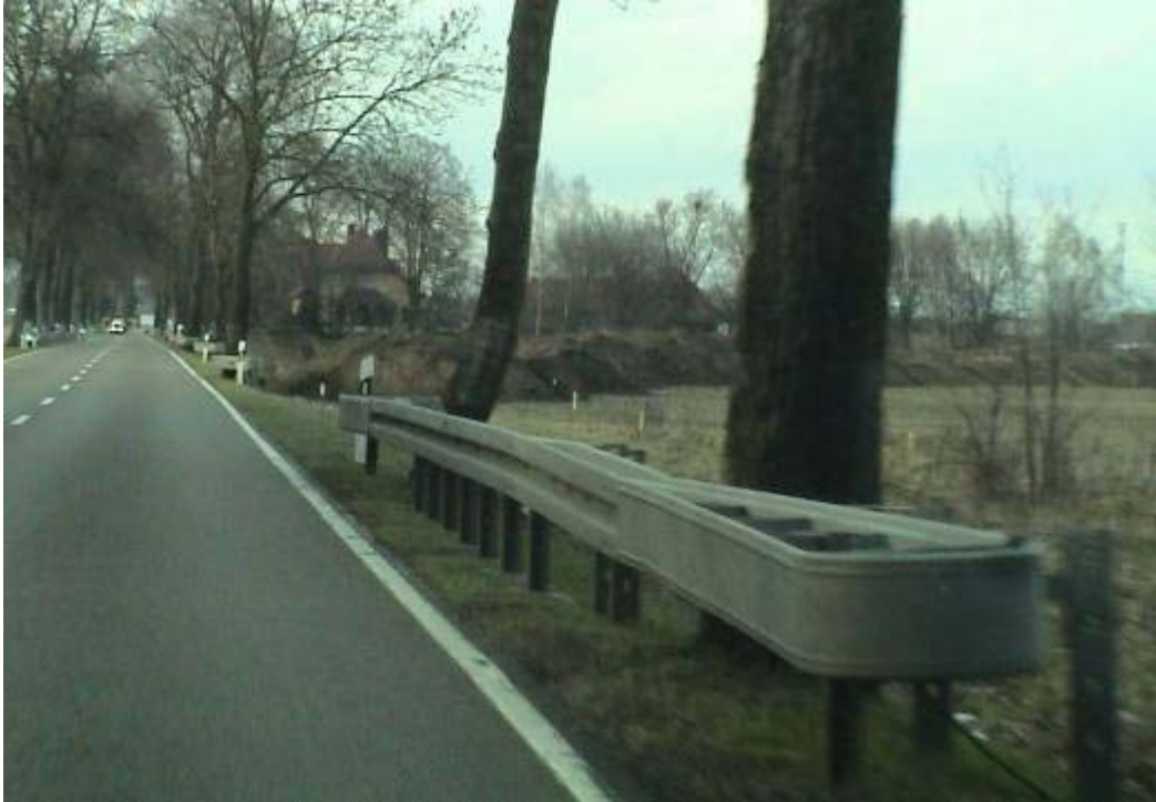
Figure 11 - Energy-absorbing crash barriers protecting trees
