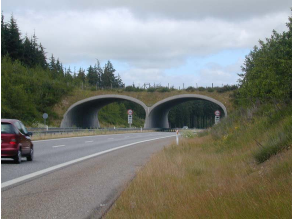
Figure 8 - The overpass at Jyske Ås, Northern Jutland. The road surface is cut into the landscape so the upper surface of the overpass is in level with the surroundings.
