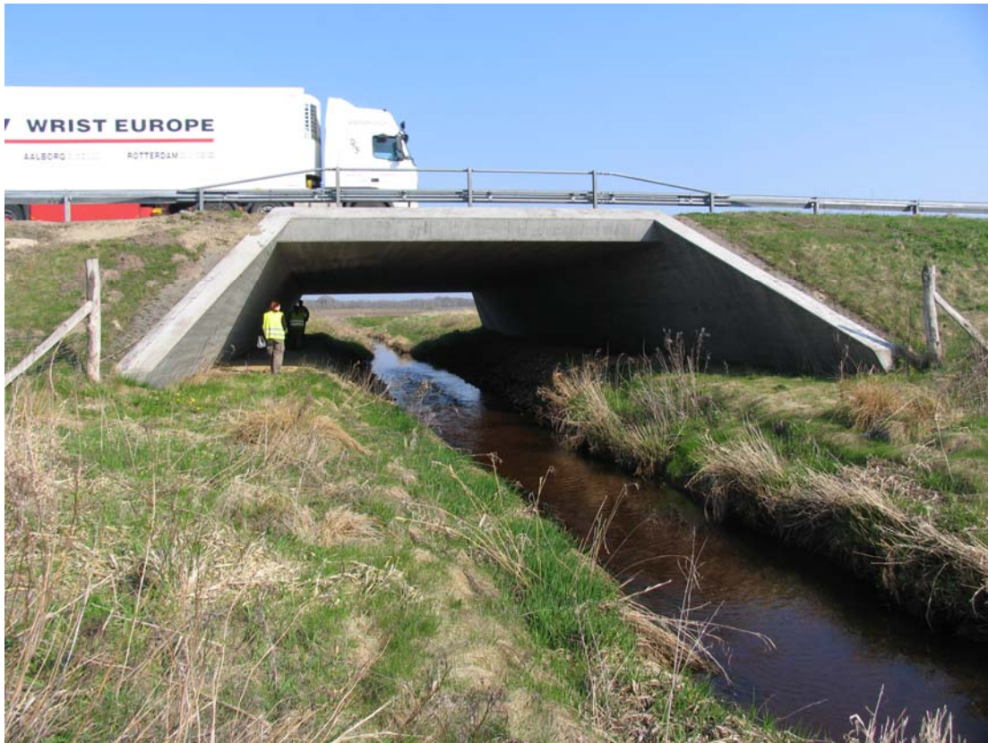
Figure 6 - Wet underpass. The fauna passage has been constructed with banquettes on each side of the watercourse. The banquettes have plane surface at the top and sloping sides towards the water.
