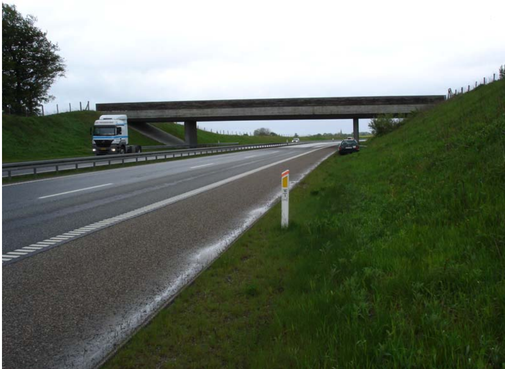
Figure 9 - Overpass at the motorway Århus - Låsby, Middle Jutland.
