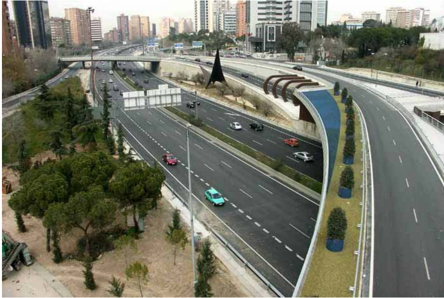
Figure 6. La Paloma interchange
