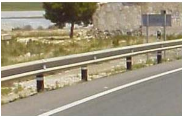
Figure 5 - Protection made of recycled rubber N344. New guardrail design.
