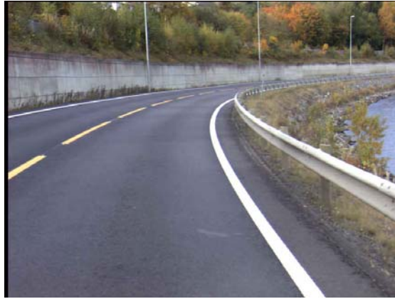
Figure 4 - Example of misplaced lighting equipment
