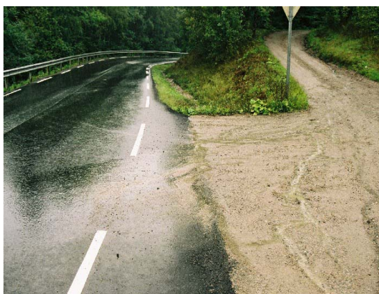
Figure 3 - Example of intersection with minor dirt road commented on after the inspection
