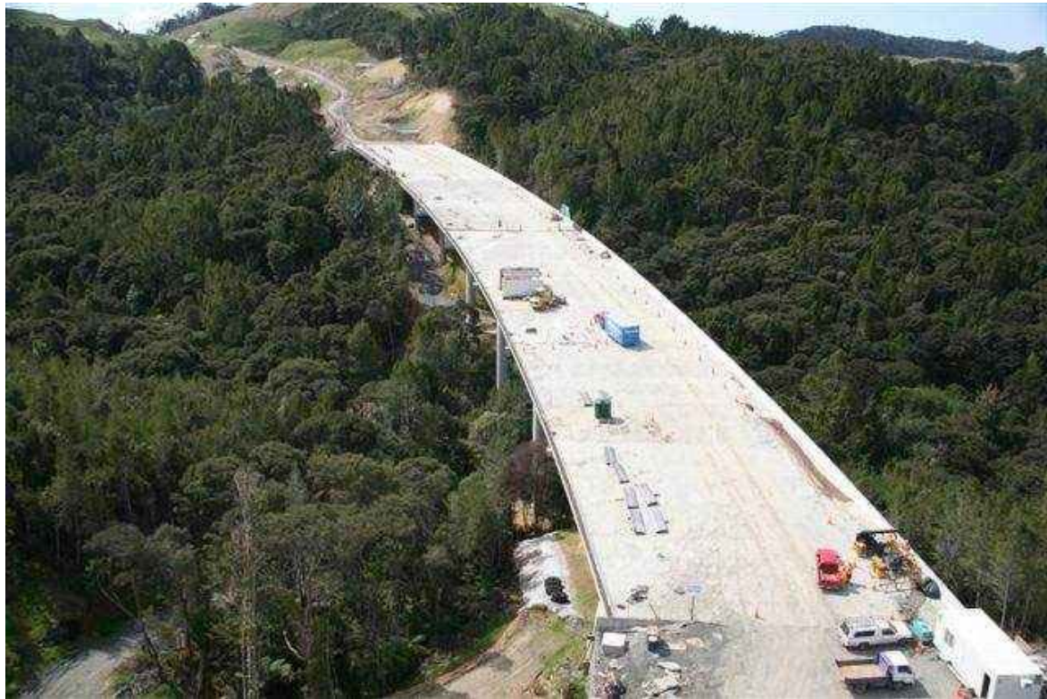
Figure 5 - Otanerua Eco Viaduct
