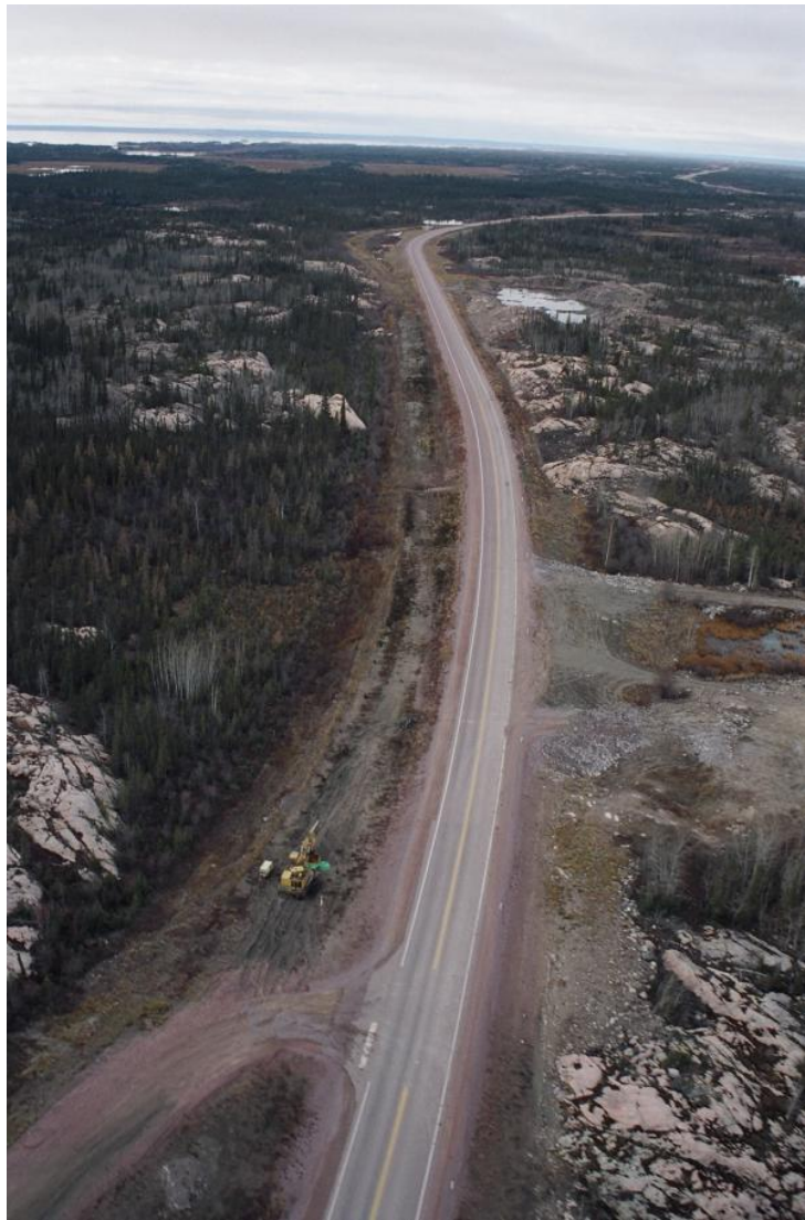
Figure 3 - Yellowknife Highway After Reconstruction
