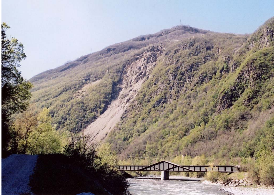
Figure 2 - View from the upstream: the bridge of the new road on the Romanche river and the Couloir des Ruines
