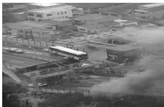
Figure 1 Damaged Highway by Great Hansin Awaji Earthquake
