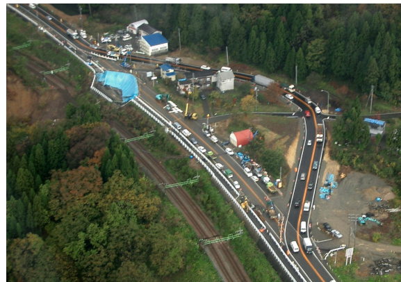
Photo 9 Detour at Tenno, national highway Route 17 [3]
