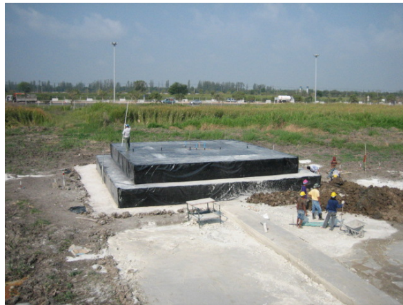
Photo 1 - Test Banking Construction
