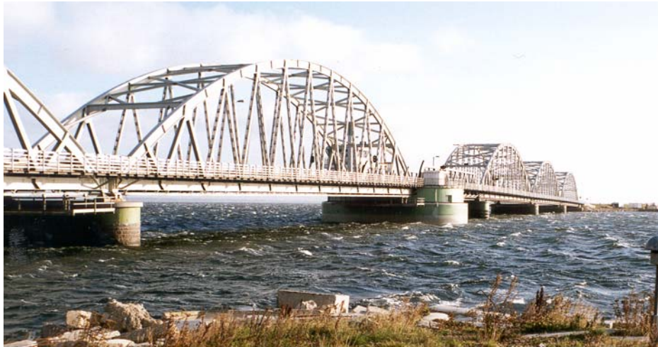
Figure 5 - Vilsund Bridge, Denmark. 5 ordinary spans and 1 bascule span.
