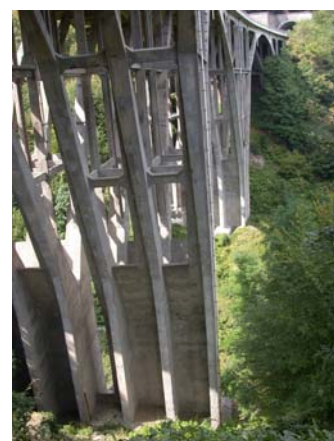
Detail of pier
