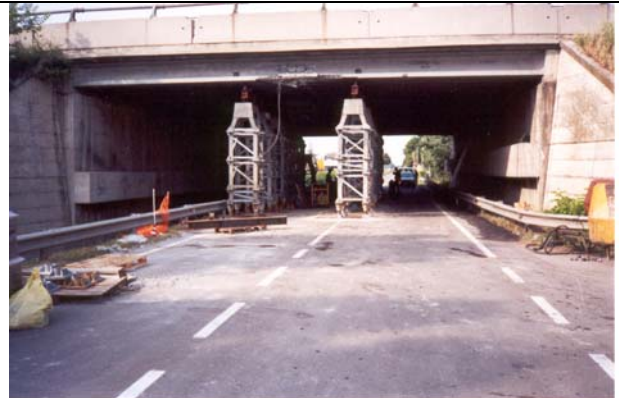
Injured structures shored by lattice steel columns
