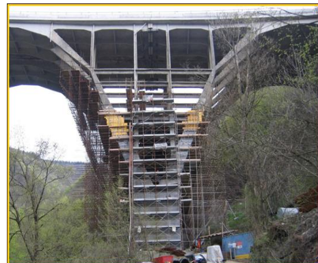
Maintenance work on bridge
