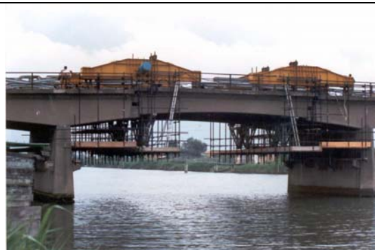
Lifting a concrete "gerber" span
