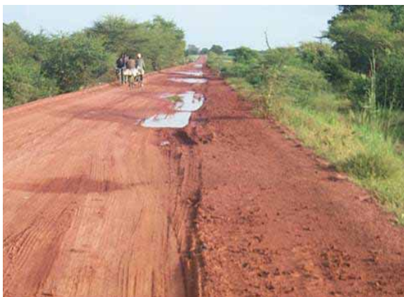
Figure 11 - Example of ruts and distortions. (Source Mahamadou OUEDRAGO, Burkina Faso)
