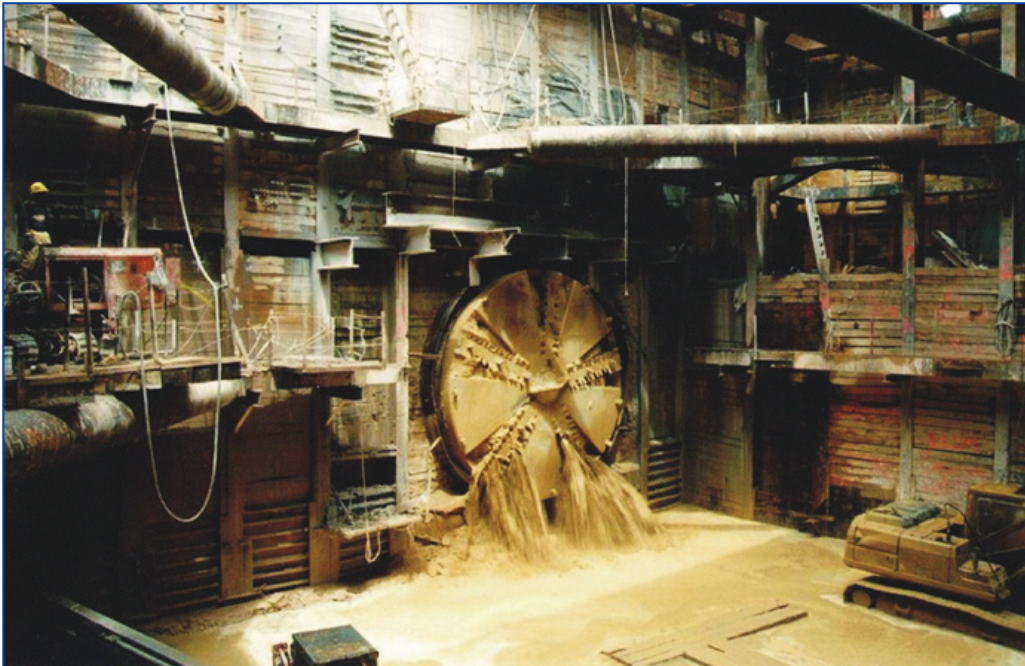
Figure 12 - Tunnel Boring Receiving/Launching Pit
