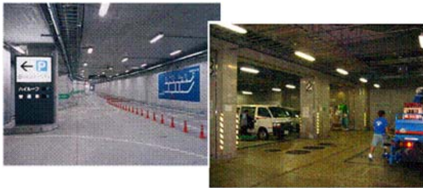
Photo 1 – Large-scale underground driveway and underground facility for loading and unloading goods (Shinagawa Intercity)
