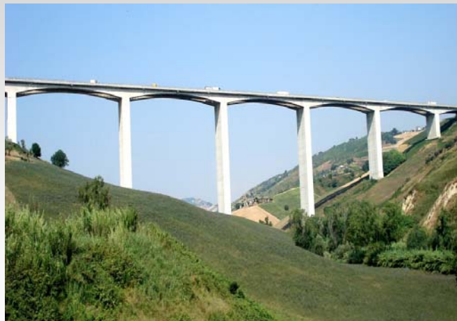
View from below (Tolaccia – box girder with monolithic piers)
