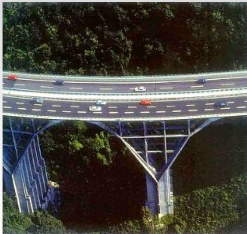
View from above (Carè e Giannelli – Arch Bridge)
