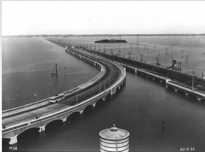
View from above (Miozzi – Masonry arch bridge)
