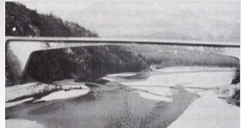
Side view (Zorzi – hyperstatic reinforced concrete frame bridge)
