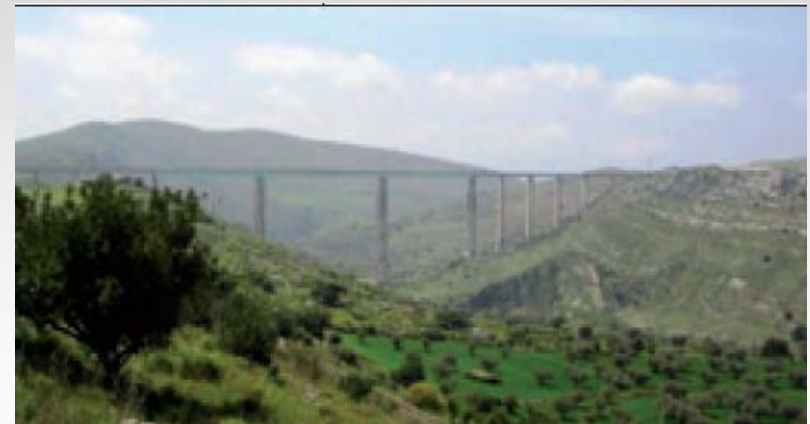
Overall view (Morandi - steel box girder spans)
