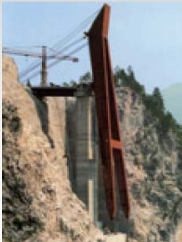
Mounting of the inclined pier (Matildi – inclined pier steel frame)
