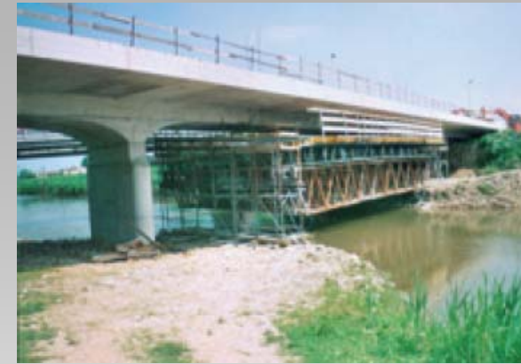
View of the deck underside
