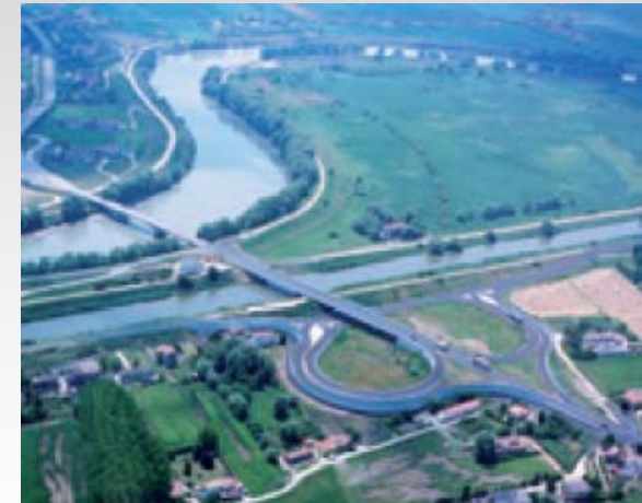
View from above (Russo e Prisco – hyperstatic reinforced concrete frame)
