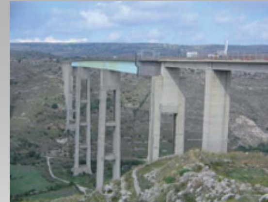
View of deck spans and piers
