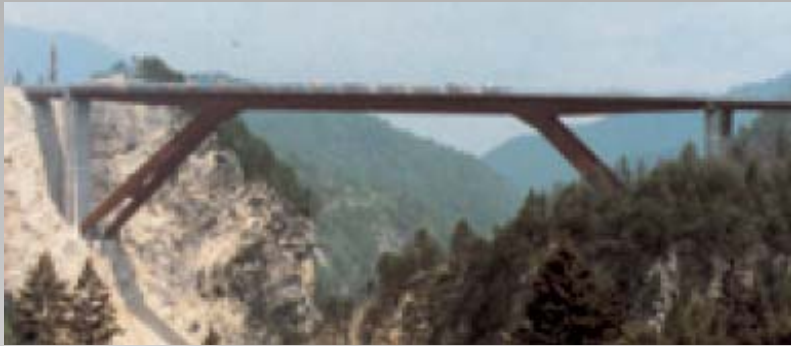
Bridge over Piave at Caralte (Belluno)
