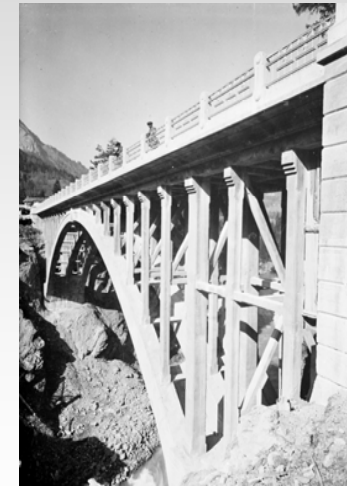
View from East abutment (Miozzi – triple arch supported-deck bridge)
