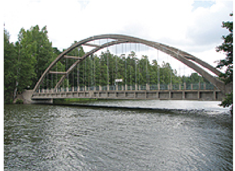
Savukoski bridge, single span concrete arch bridge (1927)
