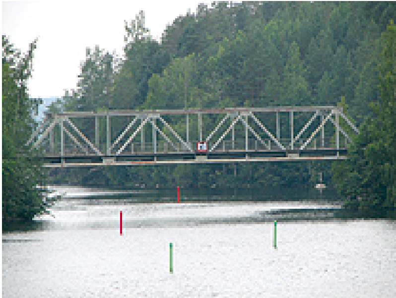
Virransalmi truss bridge (1937), use of type drawings
