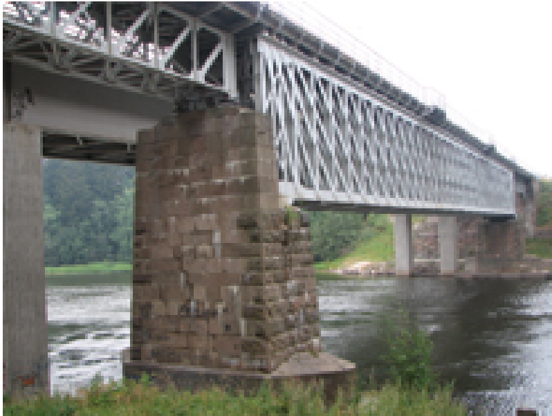
Koria steel truss bridge (1870), originally railway bridge
