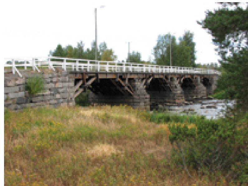
Etelänkylä wooden bridge (A-frame supporting horizontal beam, 1837)
