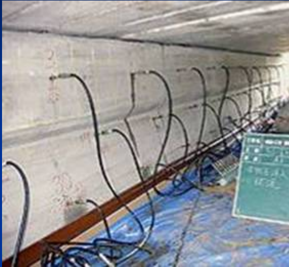
Injection of ASR-retarding agent (Sub-nitric acid lithium) into cracks
