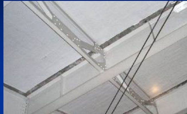
Water-proof, injection, and carbon fiber sheets
