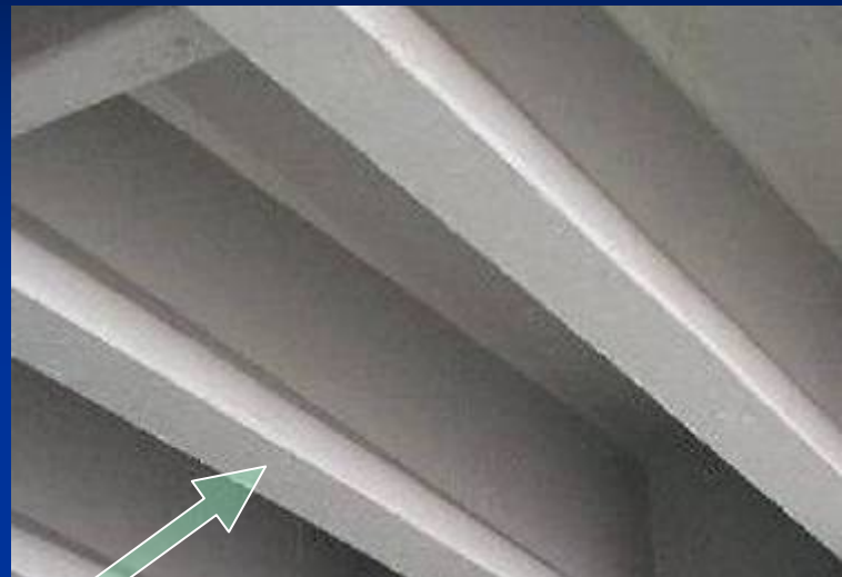
Total Repair: Sacrificial anodes and carbon fiber sheets
