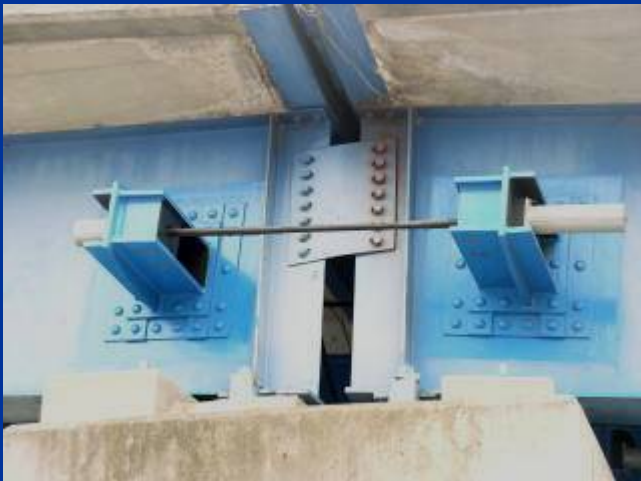
Connection of adjoining girders
