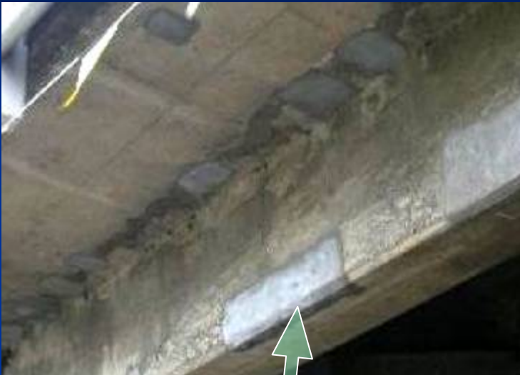
Partial Repair: Sacrificial anodes and filling concrete
