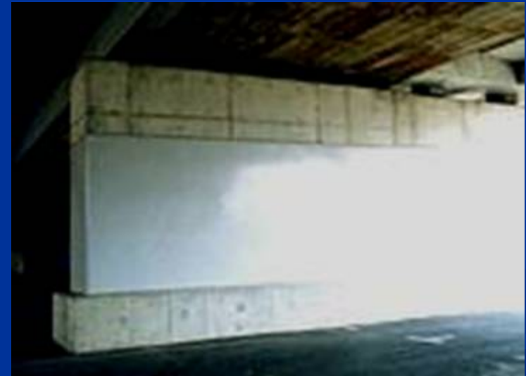
Wrapping by Carbon Fiber Sheets
