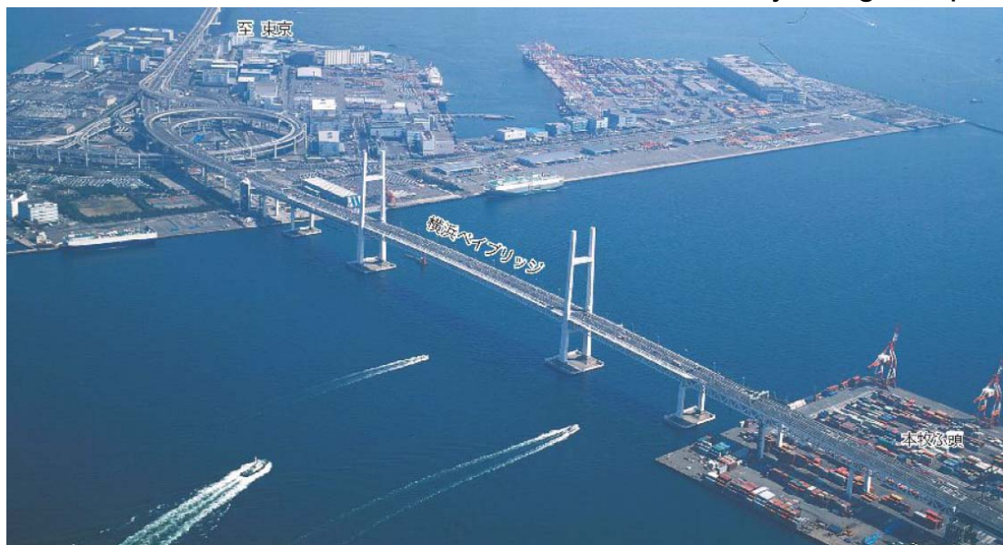
Yokohama Bay Bridge, Japan
