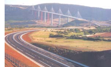
Insertion of the Viaduct in the landscape
