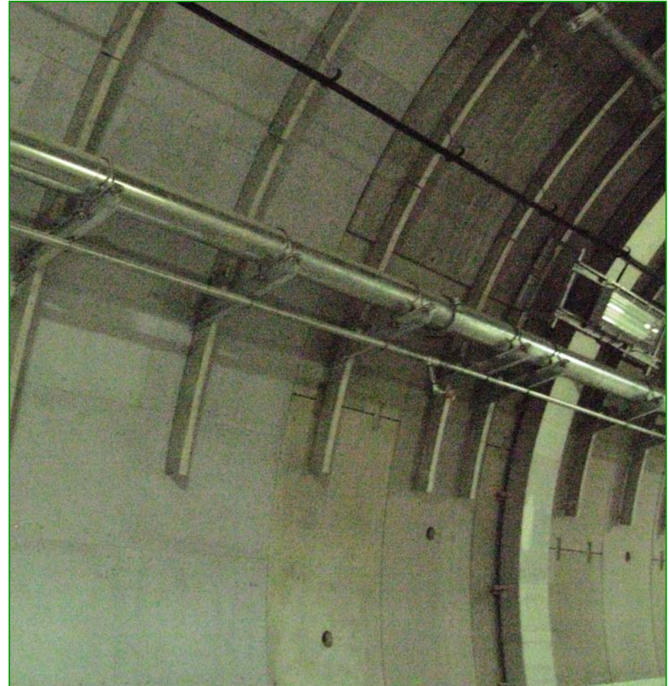
Water spray systems in a Japanese tunnel
