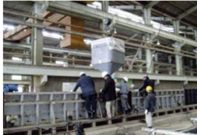
Photo 4: Coulage de poutre en BFUP Photo 4: State of placement of UFC girder
