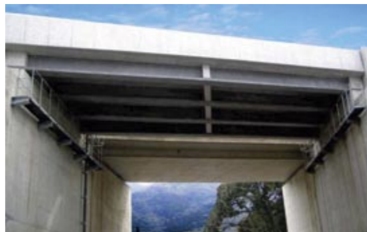
Photo 6. Photo montrant le pont achevé Photo 6. Photo showing completed bridge
