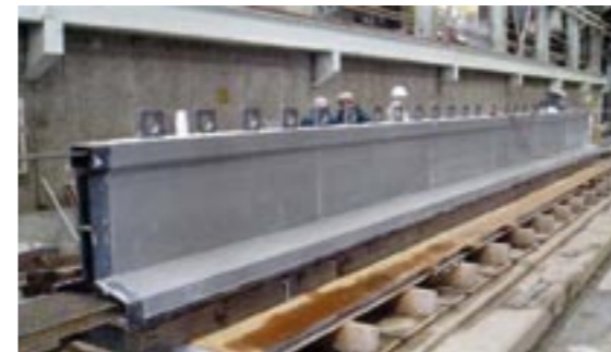
Photo 2: State when formwork was removed Photo 2 : Etat après retrait du coffrage
