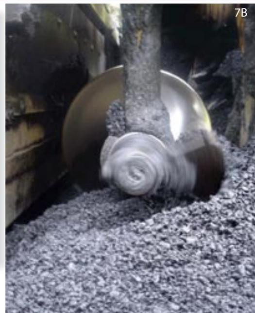
These first test sites have given full satisfaction (photos 6 and 7). The application is a classical one, i.e. using application equipment identical to that used for the control hot mix asphalts. Yet, the frequency of finisher tampers and compacting energy (number of passes) are slightly higher, in order to obtain the required level of compactness and final density. Photo 5B shows that LEA does not stick in the lorry tipper; the formation of a skin of steam condensed as fine water
